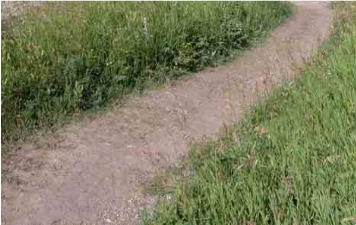
Figure 4.1 Zoom view of stabilized tread surface
