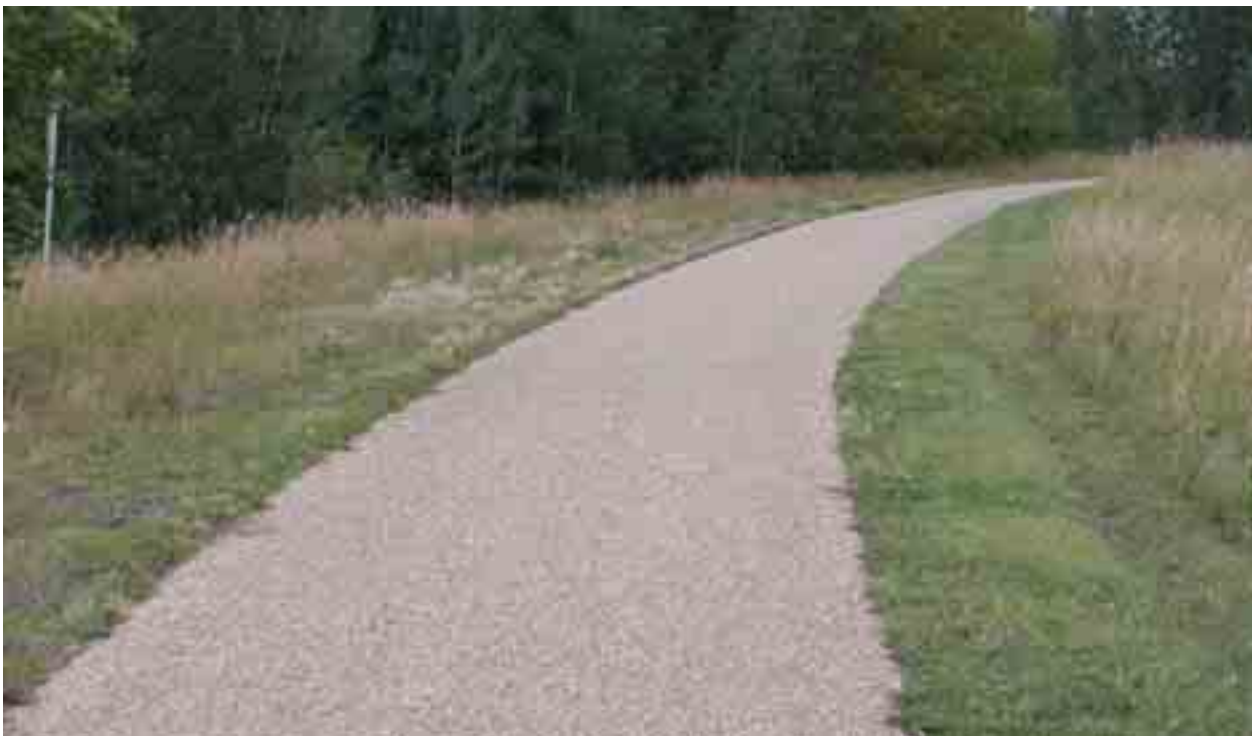
Figure 2.4 Existing asphalt with aggregate stone pathway is in good condition
