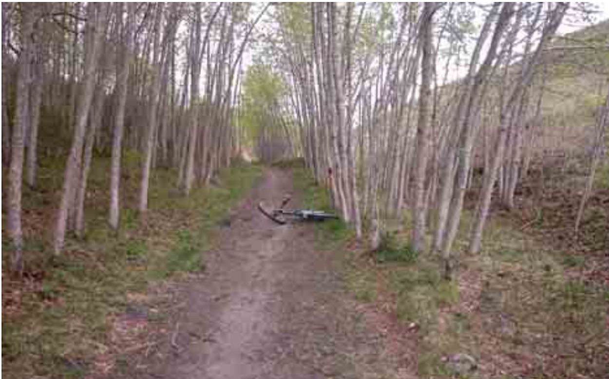
Figure 4.2 Nose Hill Park example of a stabilized tread surface
