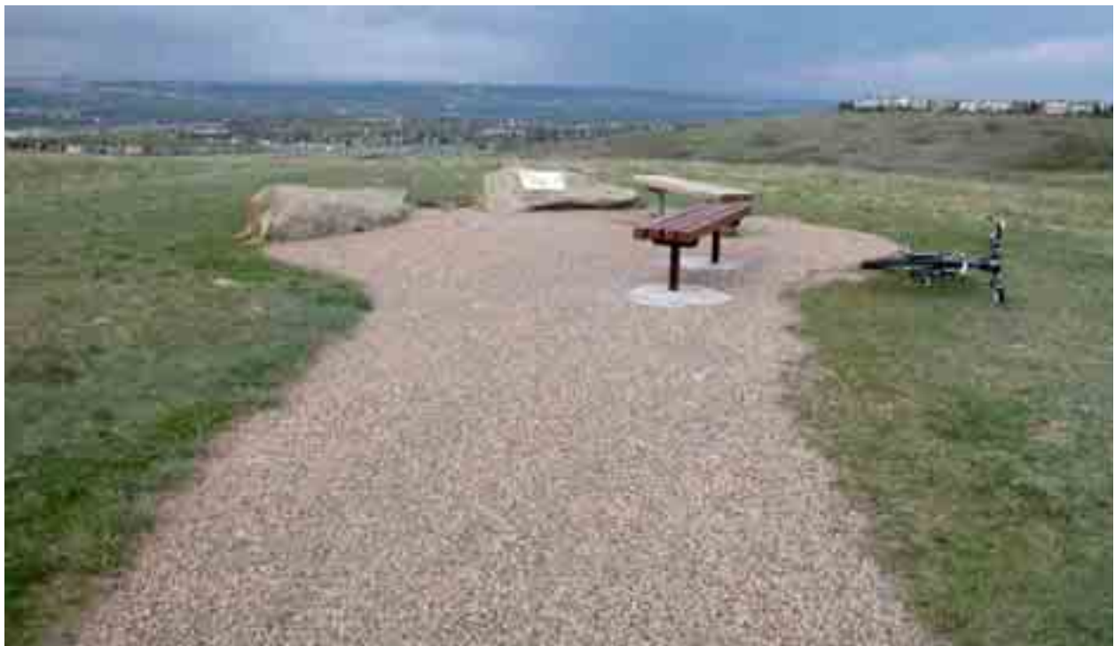
Figure 4.6 Nose Hill Park example of the asphalt with special stone aggregate surface
